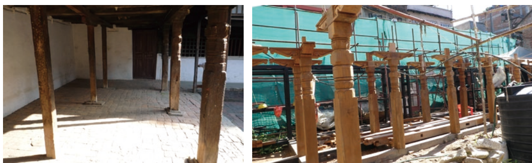
Figure 7 Changing restoration method of historic buildings: The columns with stone base ' lloham ' (left), and columns newly installed without stone base and without utilizing original materials (right). Source: ©L. Shakya
