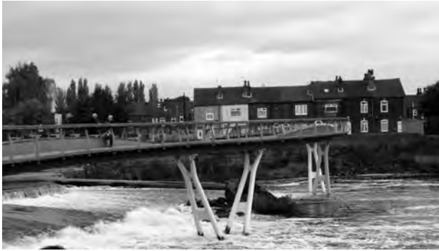
Figure 2: Footbridge, Castelford, 2010. ©L. Smith.
