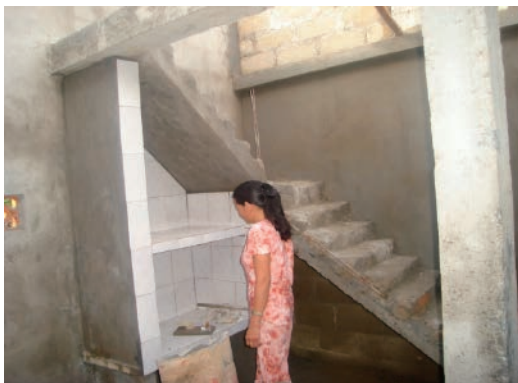
Figure 17 Two-storey pigsty (©Nguyen Thi Loc, 2008)
