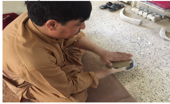
12. Polishing the tiles with a scarf to fill their holes
