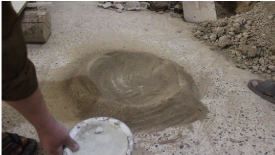
3. Mixing the ordinary soil with Barakat soil
